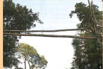
**Picture 2 and 3:** The channel sections, made of bamboo, divert water to the plant site where it is distributed into branches, again made and laid out with different forms of bamboo pipes. The flow of water into the pipes is controlled by manipulating the pipe positions.
